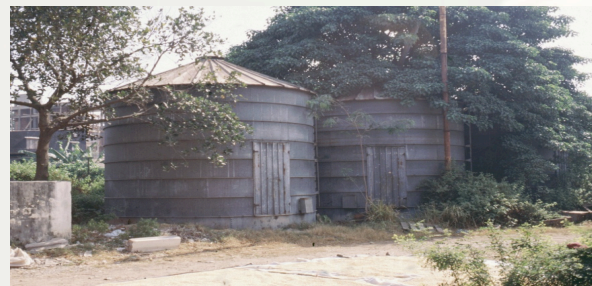
Silos: Mostly failures Technical and management problems
